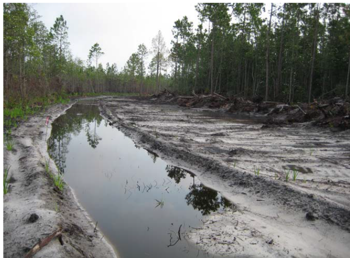
Photo 3: “Bugaboo” Line showing road trapping & channeling surface flow and berms associated with line construction.
