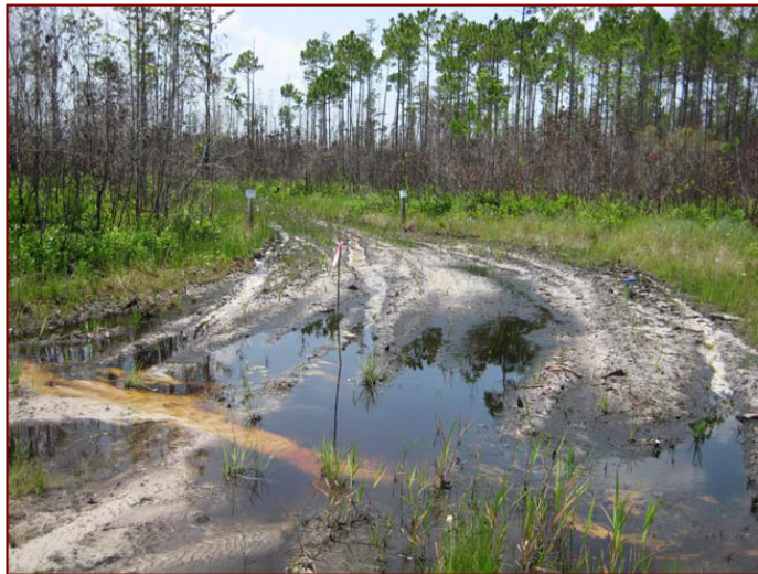
Photo 2: Service Road channeling surface flow into Road 20 ditch
