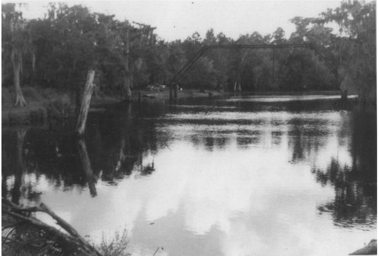
Iron Bridge: impassable by the 1940s
