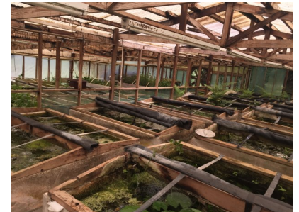
Aquatic Plant Greenhouse
