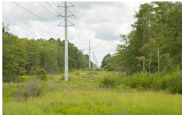
Powerline ROW through AWR-1 may facilitate solar array install onsite. (Photo by Preston Ballard)
