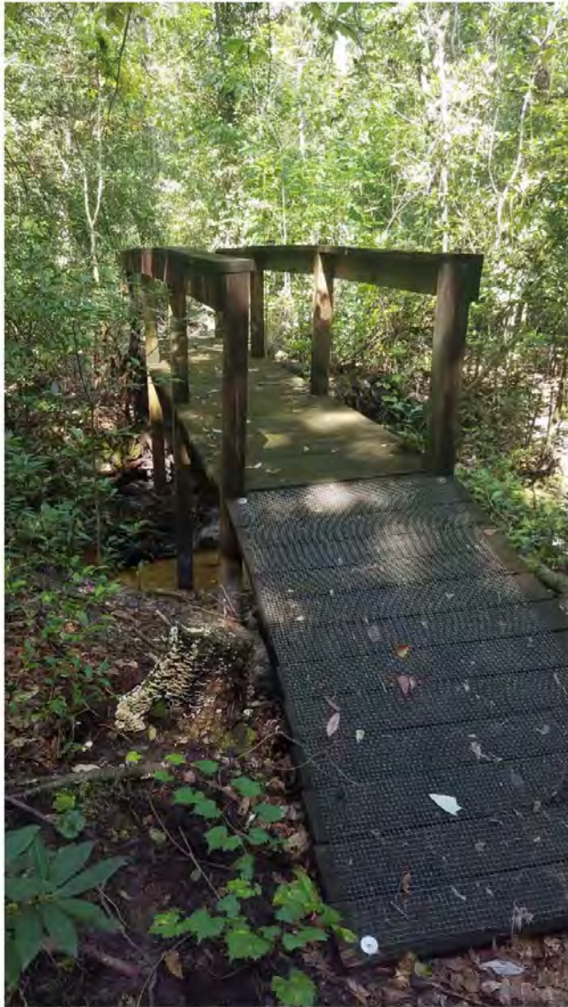
Current east bridge, photo taken facing south.
