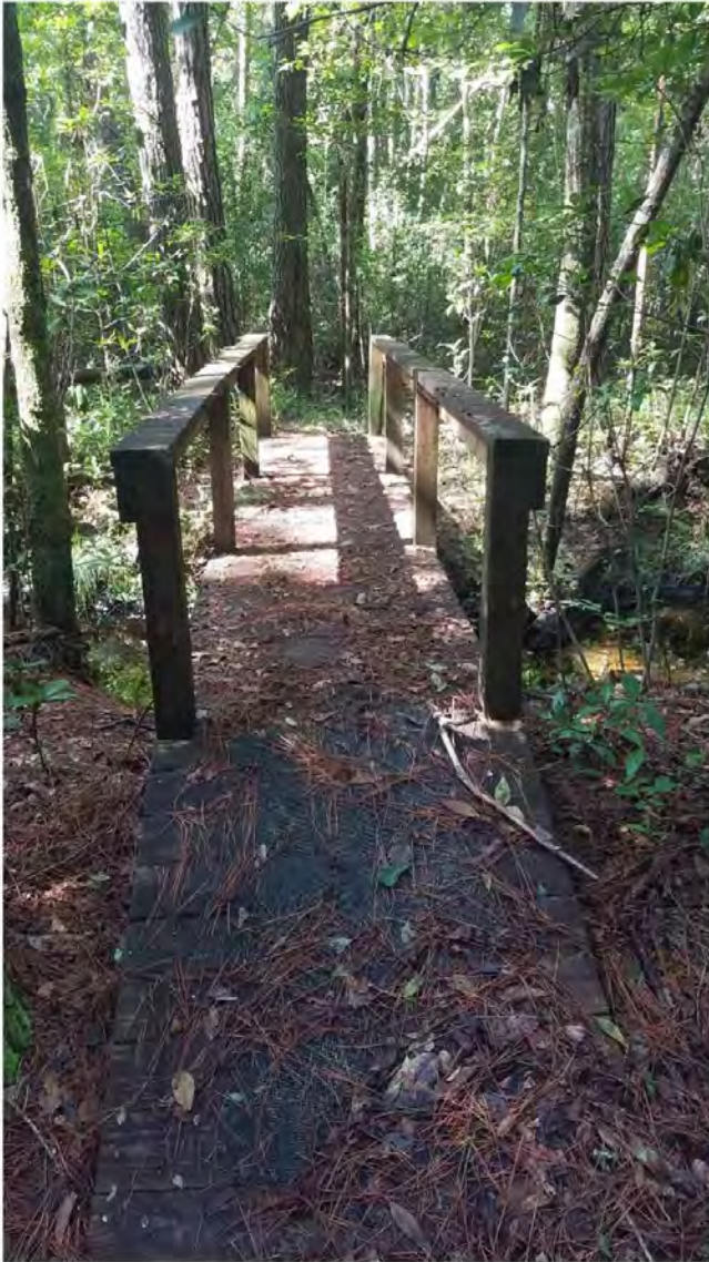
Current west bridge, photo taken south facing.
