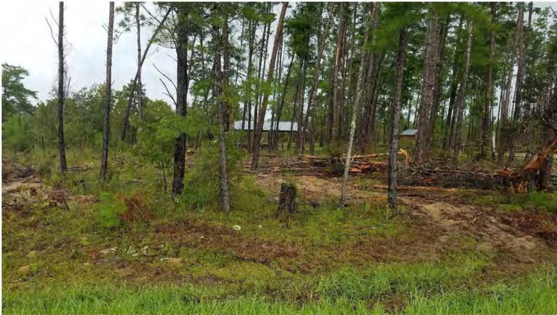
South facing photo of parking lot expansion, Lines Tract, Lake Talquin State Forest.
